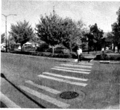
Crosswalks at Siskiyou Boulevard.
